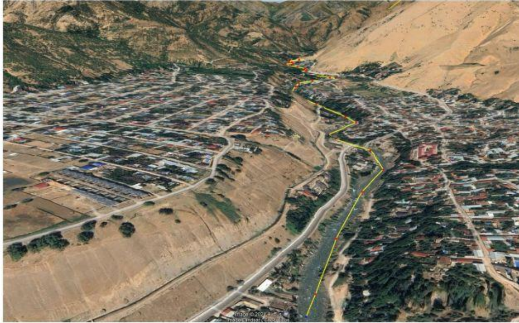
Fig. 3.5.1. Section prone to flooding near Khumsan settlement
